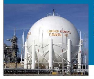
In gaseous form, oxygen and hydrogen have such low densities that extremely large tanks would be required to store them aboard a rocket. But cooling and compressing them into liquids vastly increases their density, making it possible to store them in large quantities in smaller tanks.
